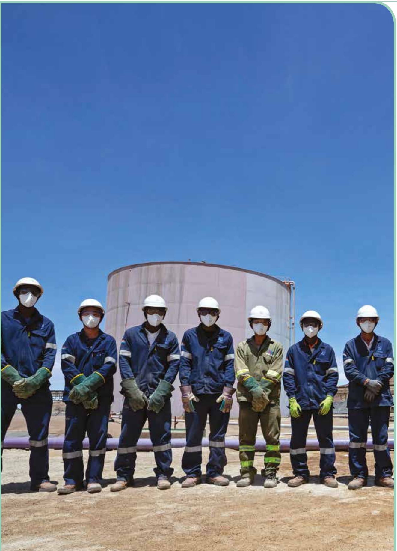
A Swakopmund-based Chinese contractor company, CNI 23, is contracted to do maintenance work on one of the acid storage tanks at the mine early in 2020, seen in the background. The company is one of many businesses supported by the mine.
