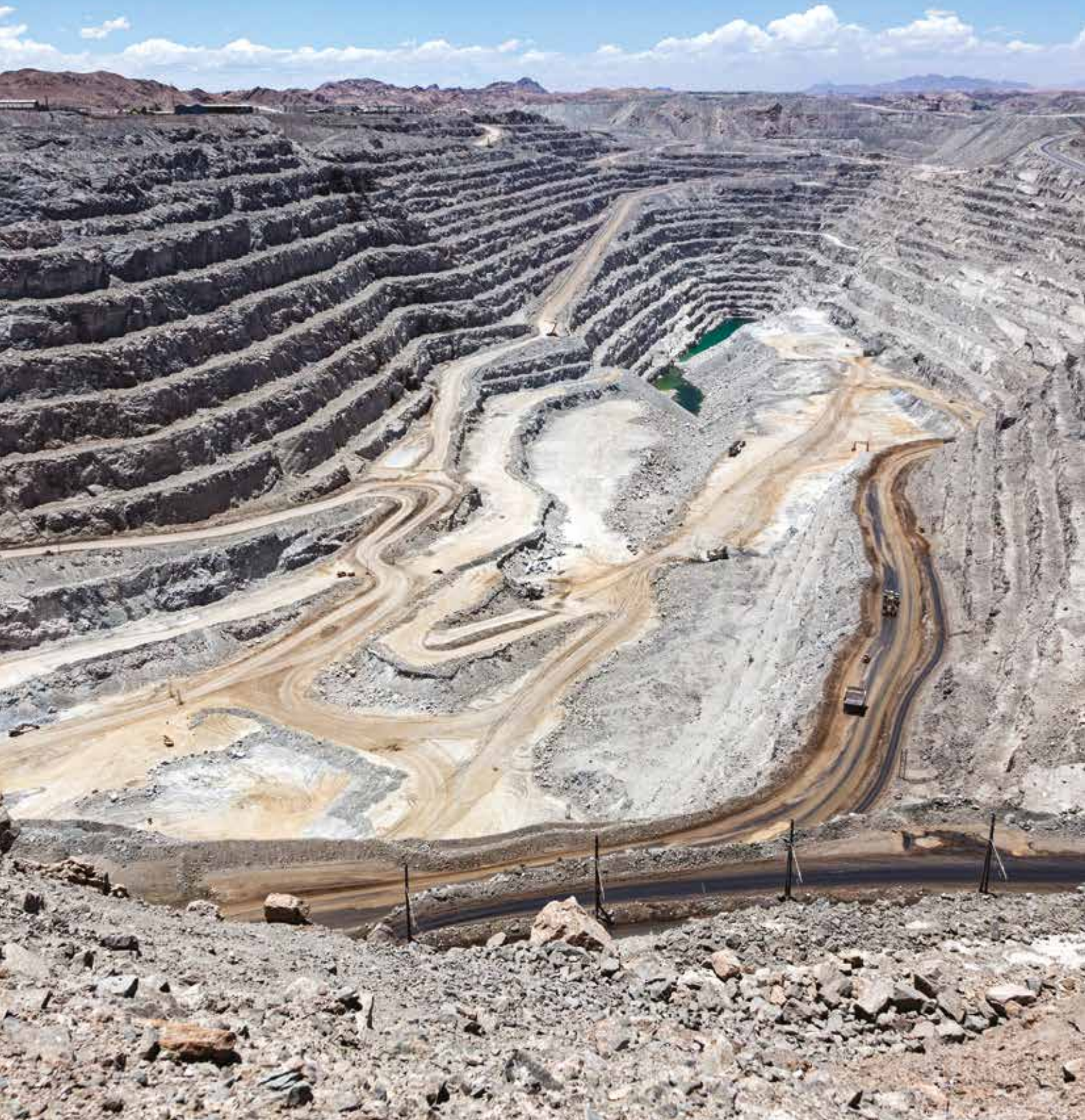
The open pit of the Rössing Uranium mine has been mined since the early 1970s with the first production of uranium delivered in 1976. The uranium located in Rössing's mining licence area is embedded in very hard and abrasive granitic rock, known as alaskite . The open pit is currently 3 km long, 1.5 km wide and 390 m deep.
