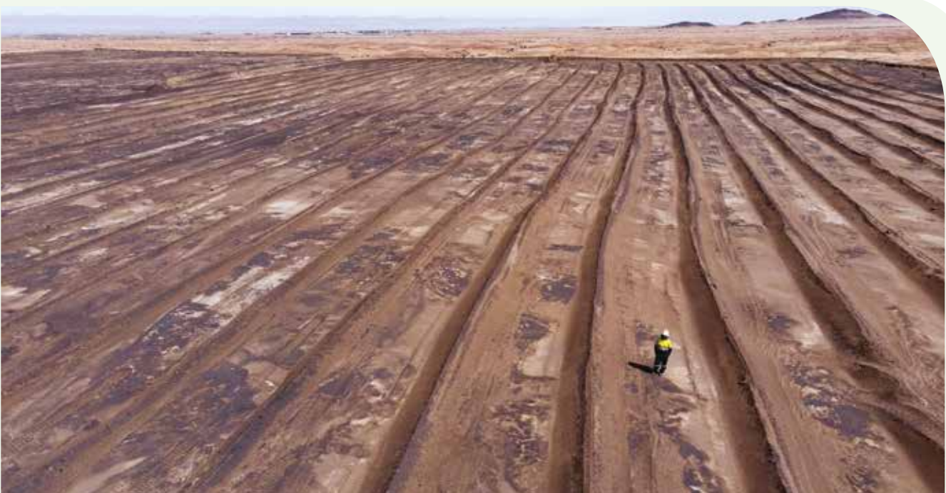
Vistorina Nangolo, Environmental Advisor: Air Quality, at the wind rows on the Tailings Storage Facility. To manage and minimise the airborne dust emission at the dry or redundant paddies, wind rows are prepared using heavy equipment. These wind rows are of a specific design, which break the prevalent air flow over the paddies, and therefore help prevent dust from getting airborne easily.
